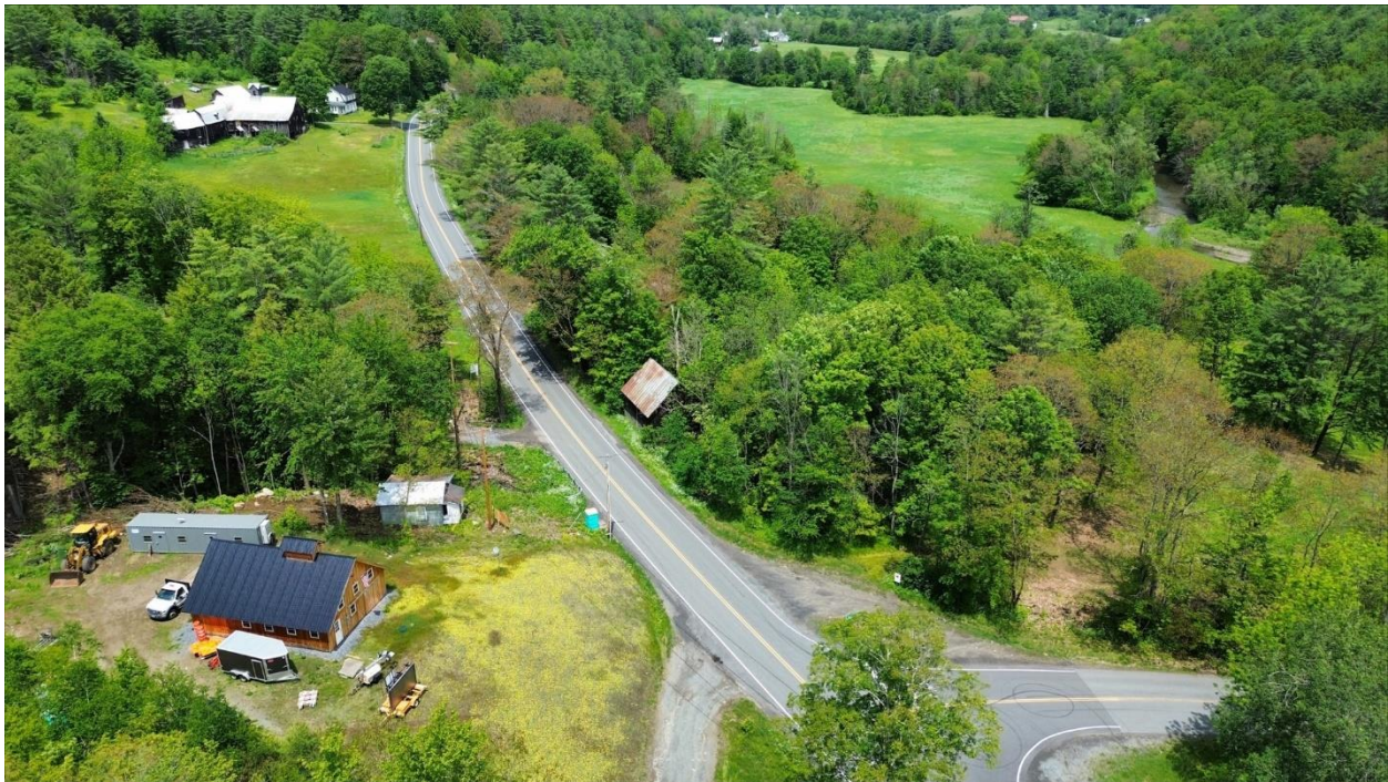
Aerial view of existing culvert conditions
